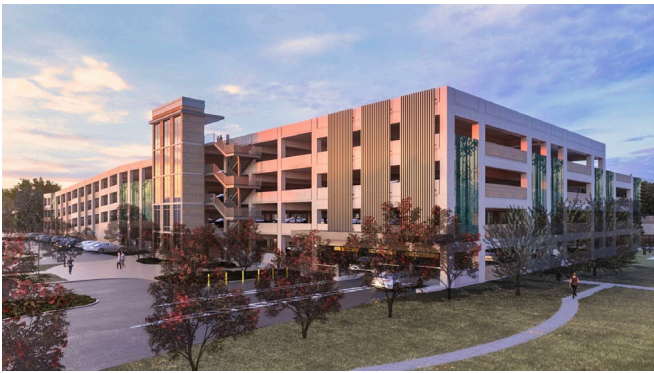
Parking Structure 7 | Aug 2025
